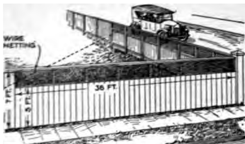
The Possibility of Accidents at a Street Crossing was Greatly Reduced by Substituting Wire Screening for Wood in the Upper Part of the Fence
